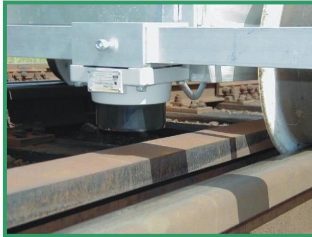
Figure 24: Detection of guard rail using inductive proximity sensor
