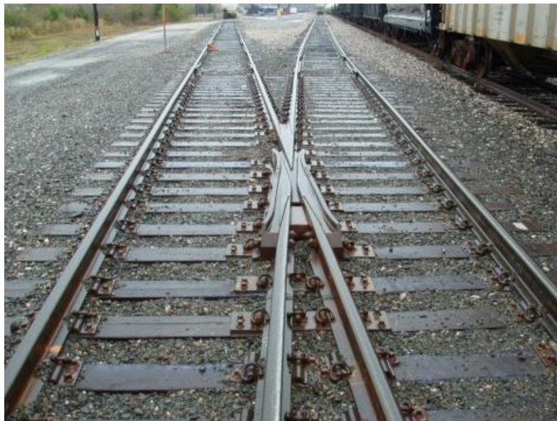
Figure 21: Switch with "self-guarding cast manganese" frog without guard rails [13]
