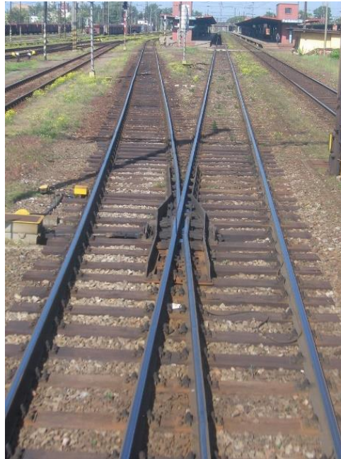
Figure 22: Switch with movable frog without guard rails [14], [15]
